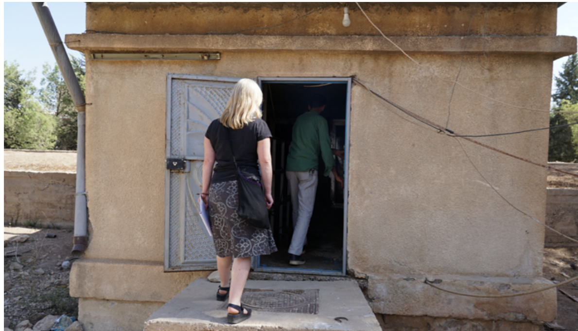
Viewing the work W4R supported at Amude Water Station
